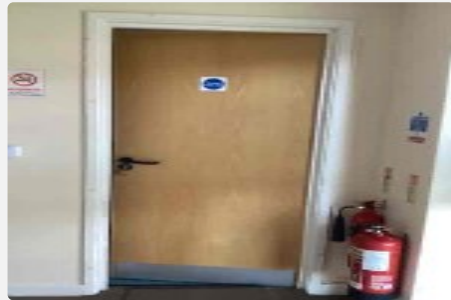
Located in store next to front entrance
